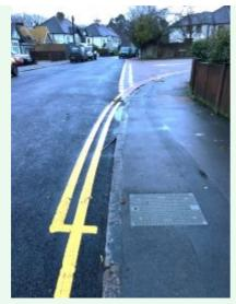
contractor didn't have red thermoplastic lining available and so thought it would be best to temporarily use yellow lining to avoid cars parking in the location. The issue has been raised with the contractor to re-attend and a follow up date to be scheduled to put the correct lining down.
